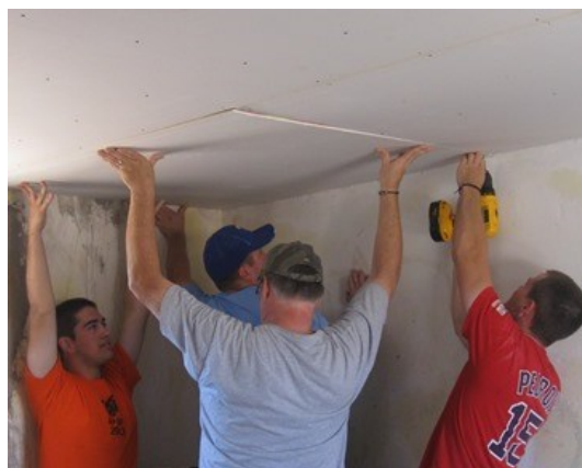
Above: The building that is being transformed into a cafeteria. Below: Team from Dunntown Advent Christian Church putting up drywall.
