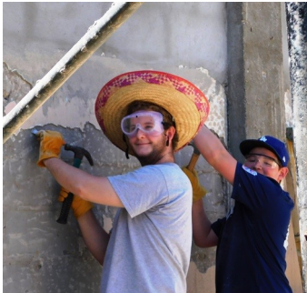
Above: Jonathan and Arroyo prepare the church wall for new stucco. Right: The new entrance roof to the youth center
